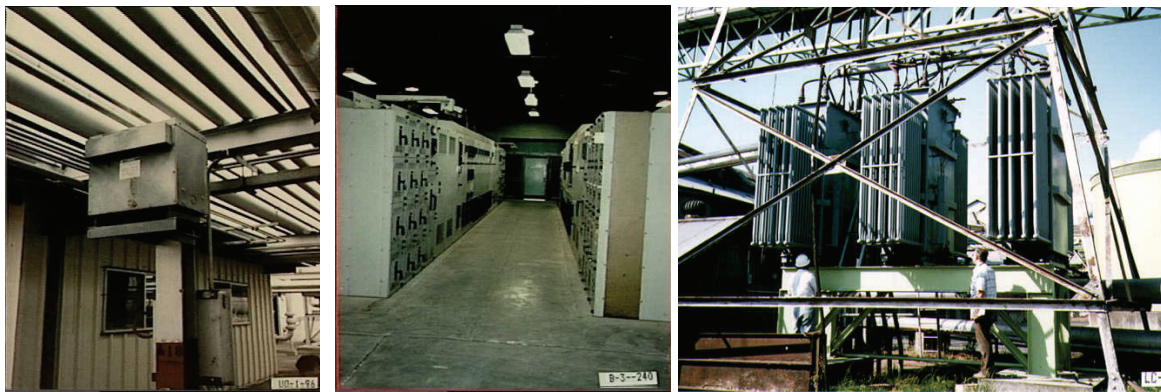
Figure 1. Some varieties of transformer: (a) 100 lb, 480/120V column-mounted, (b) 2400/480V transformers and attached switchgear
